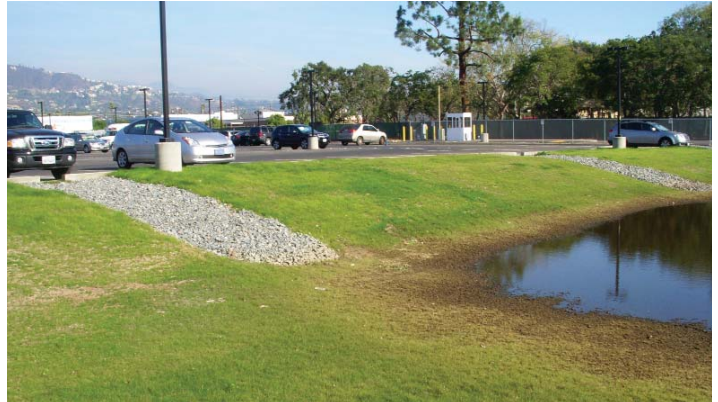
Newly seeded native grasses surround bioretention pond that captures stormwater from Burbank parking lot.
