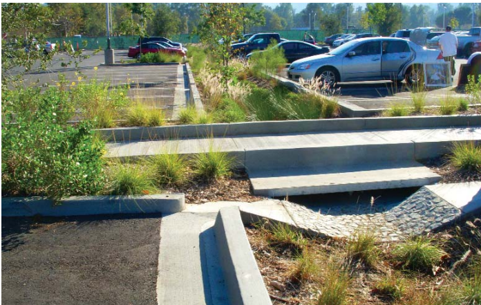
Recently constructed LA Zoo parking complex incorporating stormwater management through the use of bioswales.
